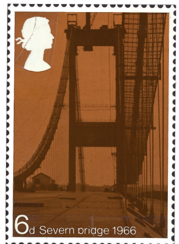
Severn Bridge during construction
